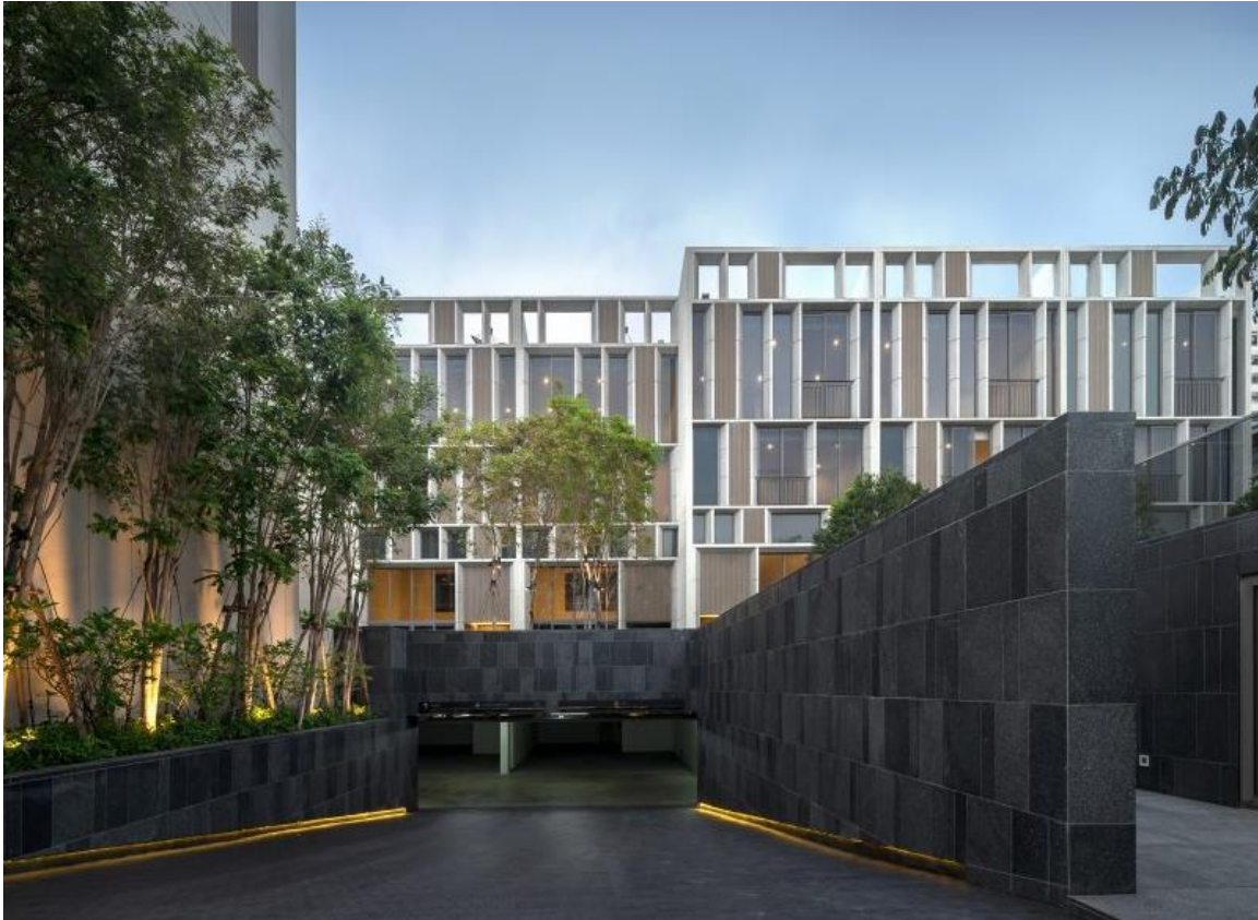
DRIVEWAY KLEADING TO BASEMENTS AND SERVICE TUNNEL
